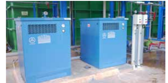
Figure 9 - Blower Package with Hood for Aeration in Waste Water Treatment Plant
