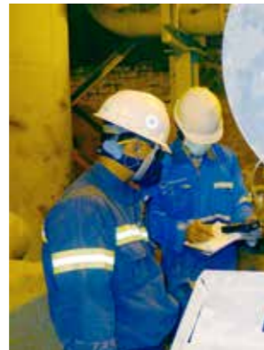
On-Site Troubleshooting & Maintenance
